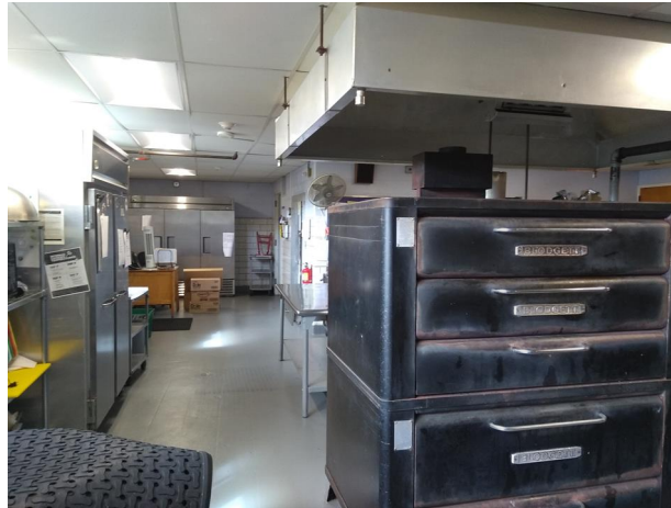
26. Kitchen equipment is very old and inefficient.
