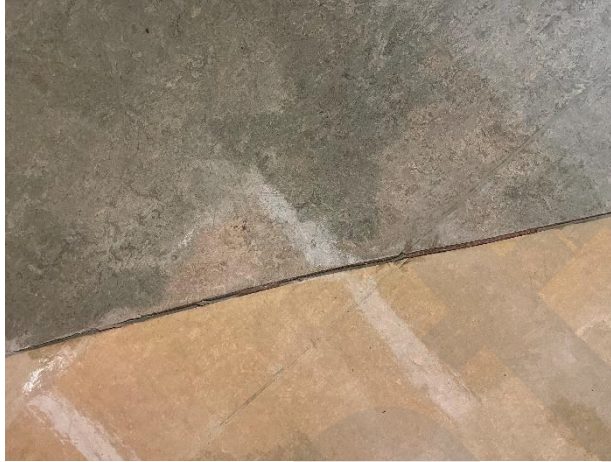
8. Some floor joints at natural linoleum are damaged.
