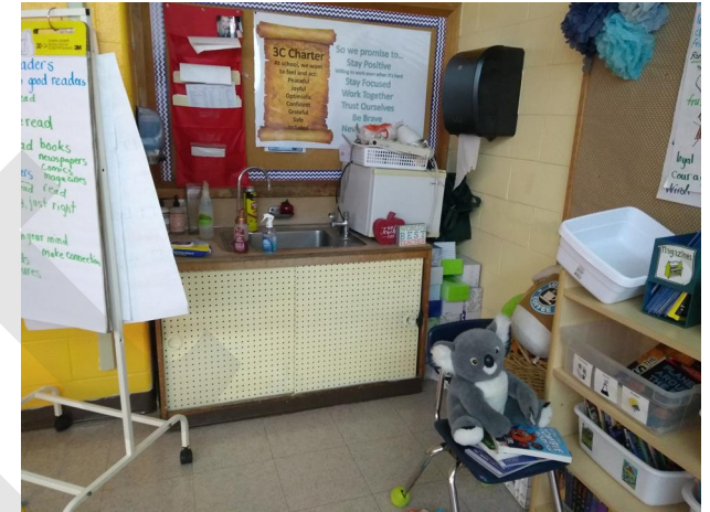
21. Classrooms have outdated sinks that do not meet AAB accessibility requirements.
